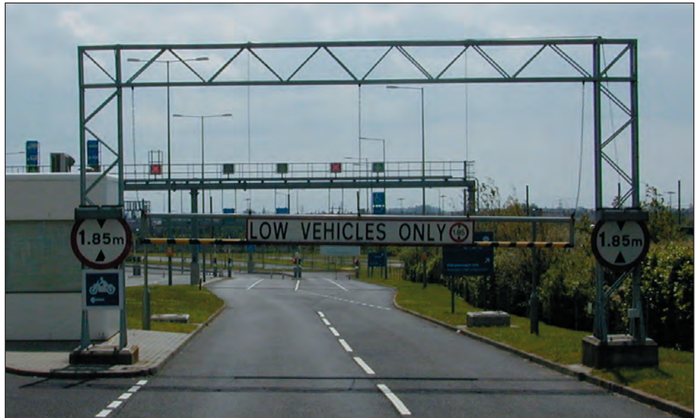
This simple poka yoke device ensures that no vehicle that is too high for the Channel Tunnel shuttle train can ever attempt to enter it
